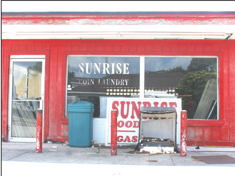
Bo Bayer said that for two days recently, an overpowering odor was coming from a building formerly occupied by Sunrise Laundry.
